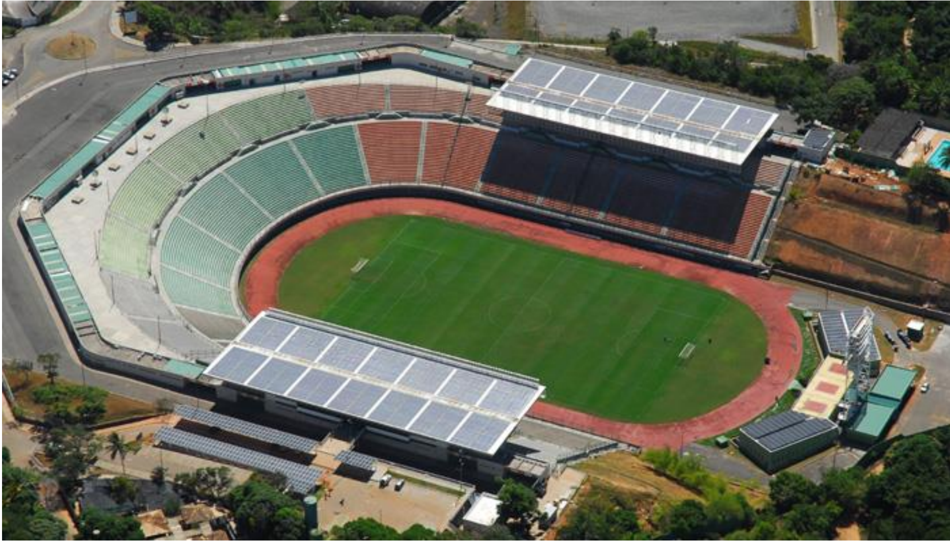
Pituaçu Solar, 400 kW – COELBA, Salvador-Bahia, 2012
